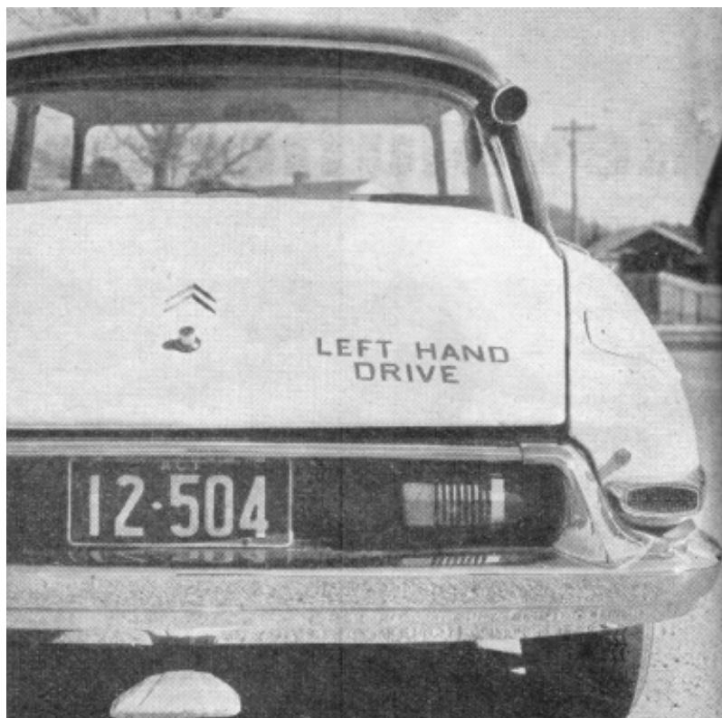
Car carries no name tag, only Citroën's chevrons. Sloping back hides huge boot. Lights on turret top are trafficators.
