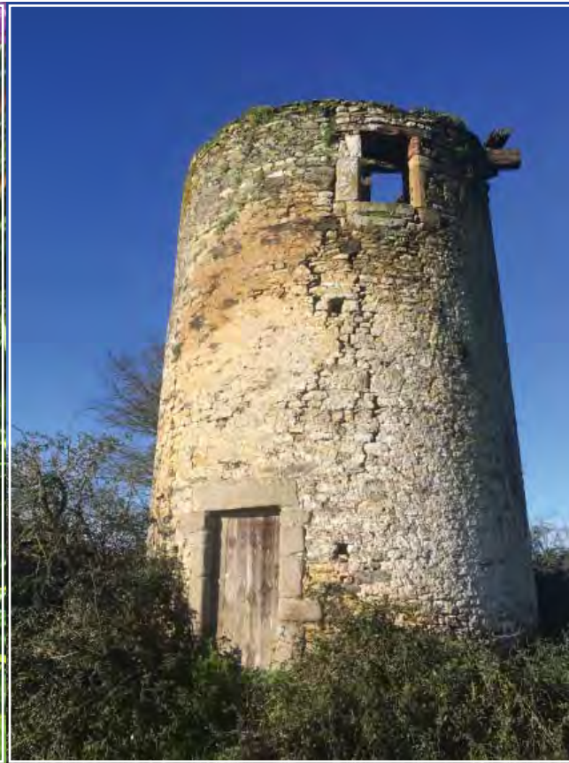
1660 windmill tower. Can you spot the date of construction ?
